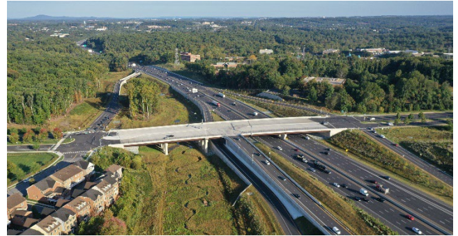
2021 Overall Project Achievement Award | Over $15 Million I-270 At Watkins Mill Road Interchange (Transportation) MDOT SHA District 3 | Wagman
