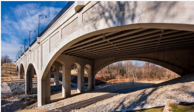
2022 Project Achievement Award | Greater Than $15M Edmondson Avenue Bridge Replacement (Transportation) Baltimore City DOT | JMT
