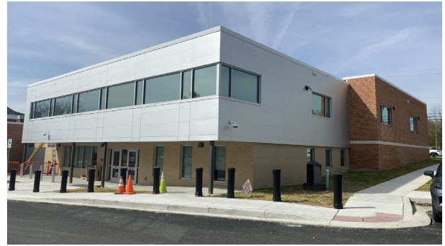
2023 Overall Project Achievement Award | Government: Construction value between $5 - $15 Million / Town of Bel Air Town Hall & Police Department / Town of Bel Air Departments of Planning & Community Development and Public Works | DFI
